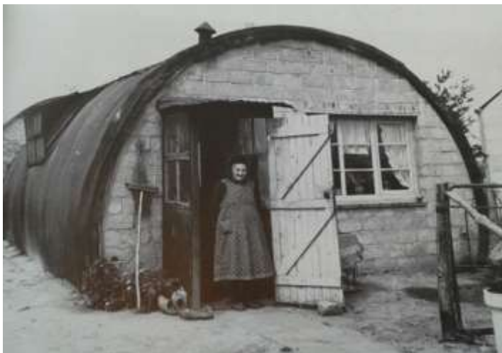
Figure 4 Temporary house in Eede
